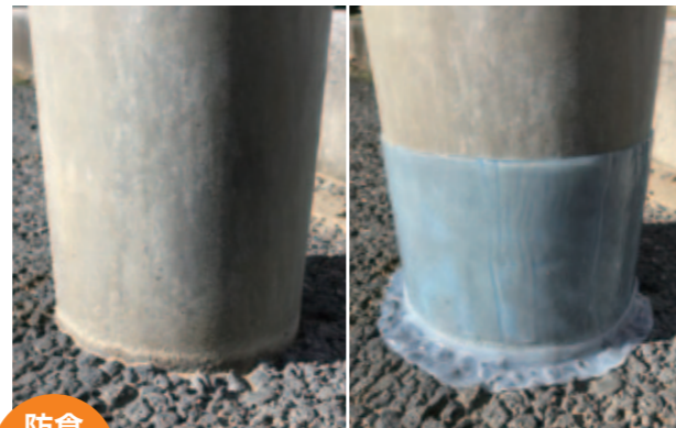
防食 Anti-corrosion 管柱地際の防食 Corrosion protection at the pipe column bases
