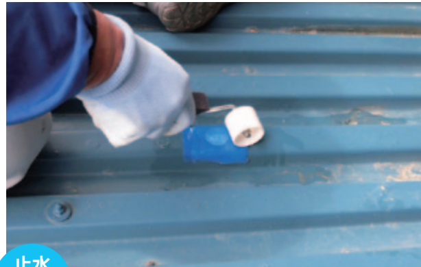
止水 Water stop 折半屋根の漏水補修 Corrugated roof water leakage repair
