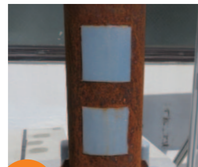
防食 Anti-corrosion 鋼管柱の表面防食 Corrosion protection of steel pipe columns
