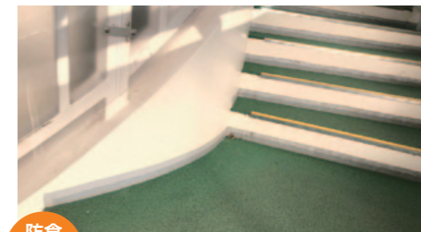
防食 Anti-corrosion 横断歩道橋の防食 Corrosion protection of pedestrian crossing bridge
