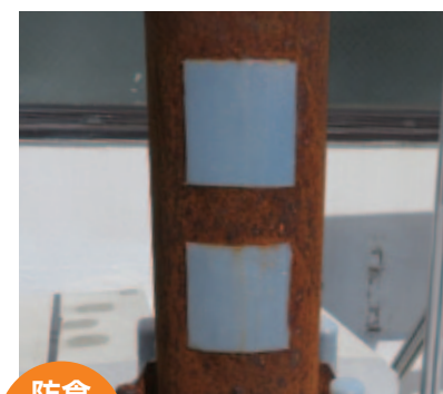
防食 Anti-corrosion 鋼管柱の表面防食 Corrosion protection of steel pipe columns
