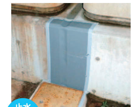
止水 Water stop 高架橋目地止水 Water stop of viaduct joints
