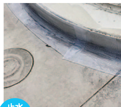
止水 Water stop 屋上防水の漏水補修 Waterproof roof water leakage repair
