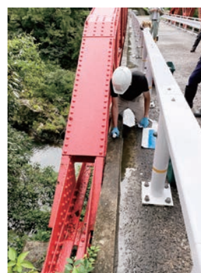
Applying “Polymer-Ace” to the bridge
