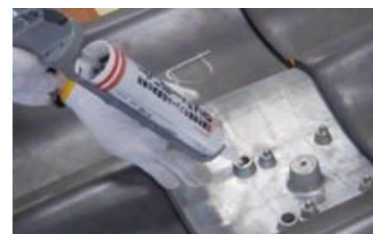
Using PV Sealant during construction work
