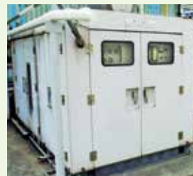
Prior to replacement
