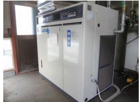
An inverter-driven compressor that can save energy (Top Runner Motors are used)
