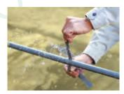
Rubber tape to prevent leakage from pipes, etc.
