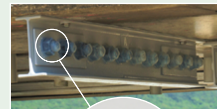
Example of actual bridge application
