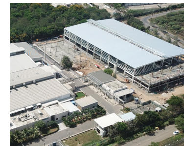
The third factory building is under construction (upper right)
